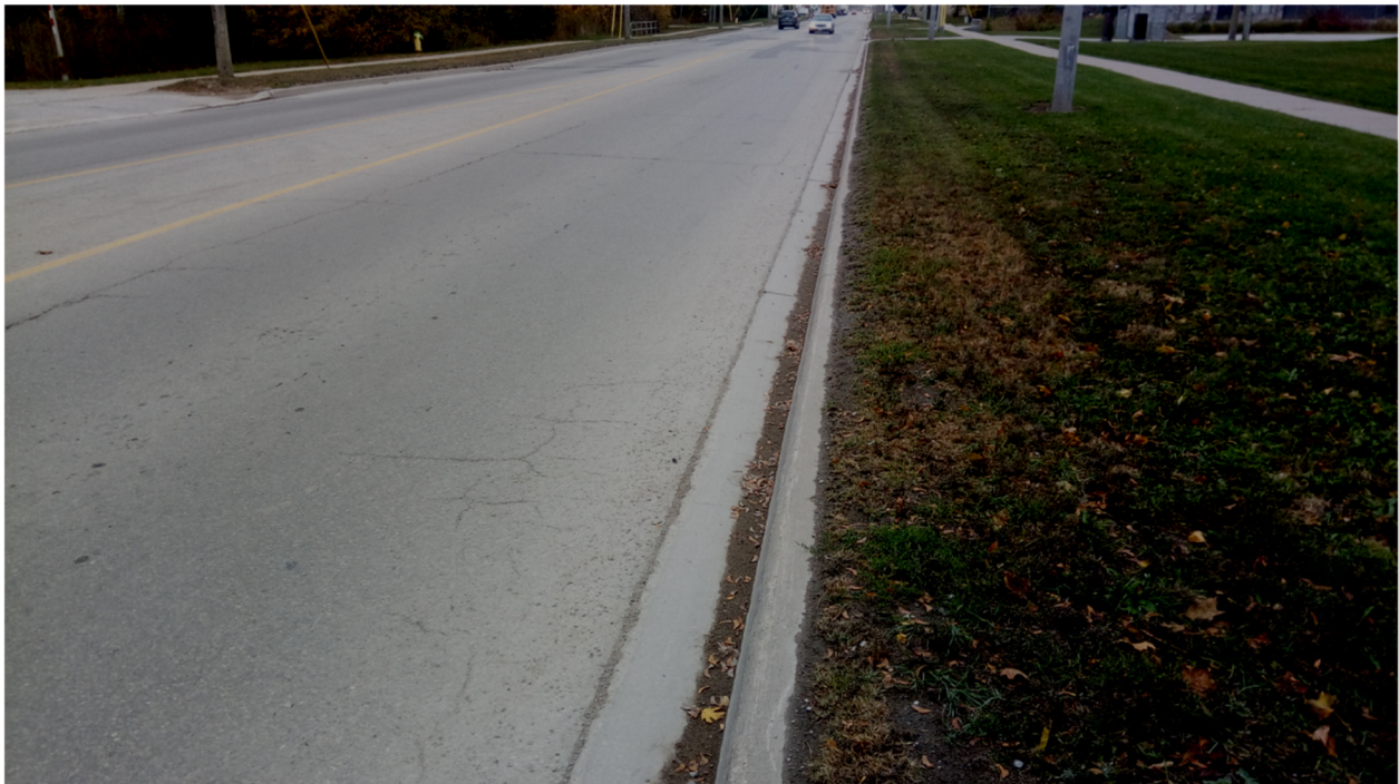
Example of a Road in Fair Condition - Tiffin Street (Wheel Track and Edge Cracking)
