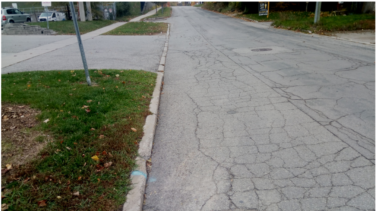
Example of a Road in Poor Condition - Maple Avenue (Map Cracking)
