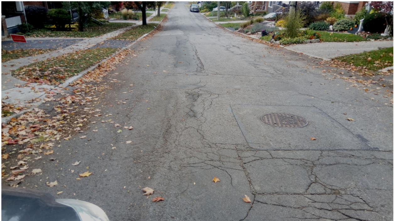
Example of a Road in Poor Condition - Mary Street (Wheel Track Cracking and Rutting)
