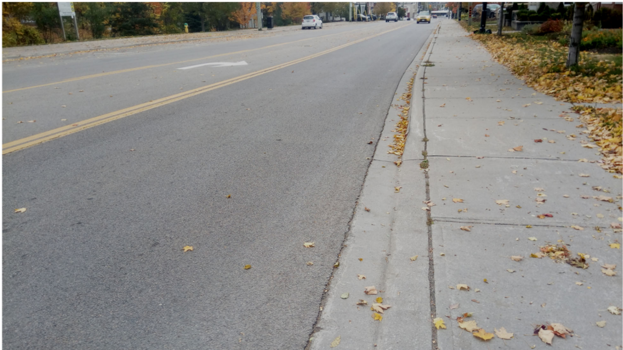
Example of a Road in Good Condition - Toronto Street (Mild Edge Cracking)
