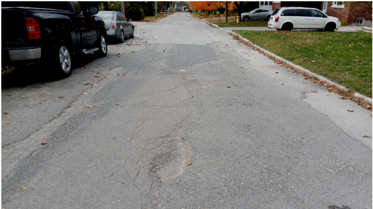
Example of a Road in Poor Condition - Thomas Street (Moderate Patching, Wheel Track Cracking and Depressions)
