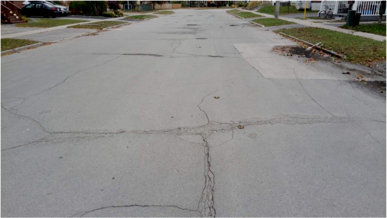
Example of a Road in Very Poor Condition - John Street (Transverse and Longitudinal Cracking, Depressions, Potholes and Rutting)
