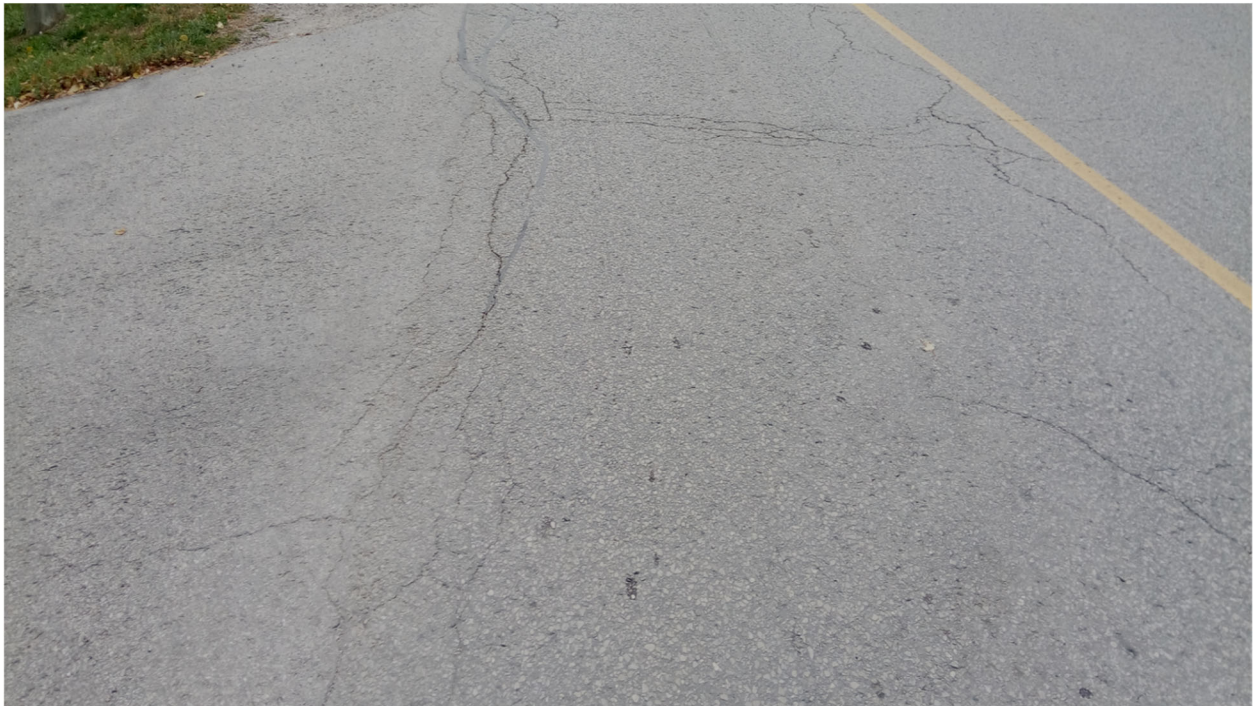
Example of a Road in Fair Condition - Edgemoor Drive (Moderate Edge and Transverse Cracking)
