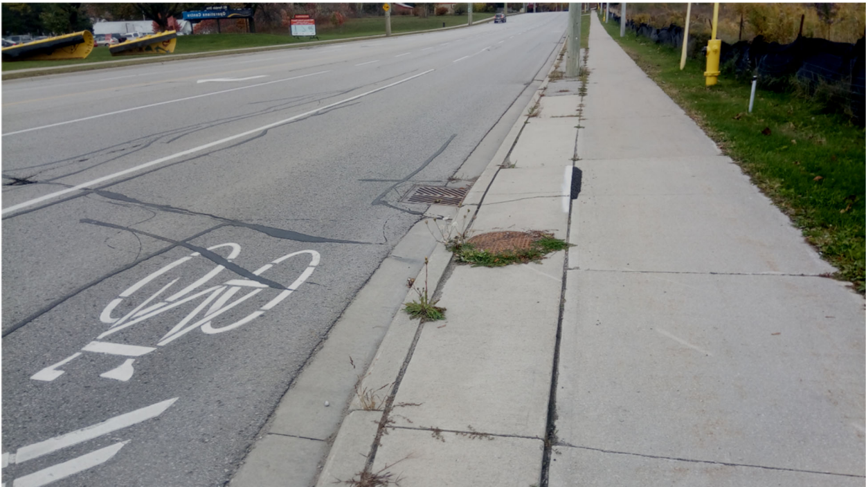
Example of a Road in Good Condition - Ferndale Road (Mild Crack Sealing)
