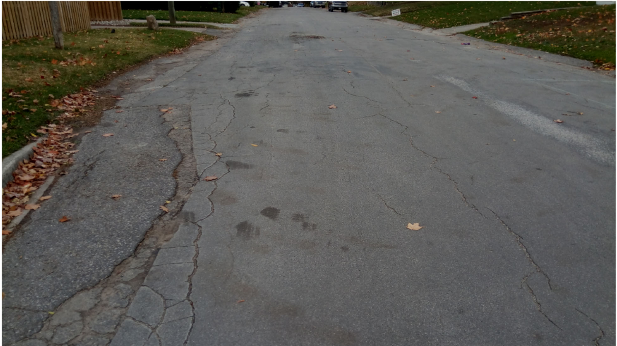
Example of a Road in Very Poor Condition - Agnes Street (Asphalt Patching, Edge and Wheel Track Cracking and Depressions)
