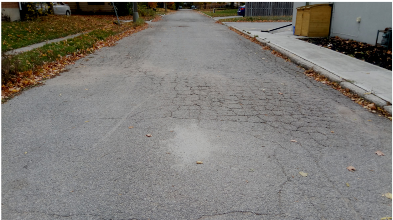
Example of a Road in Very Poor Condition - East Street (Significant Map/Alligator Cracking and Depressions)
