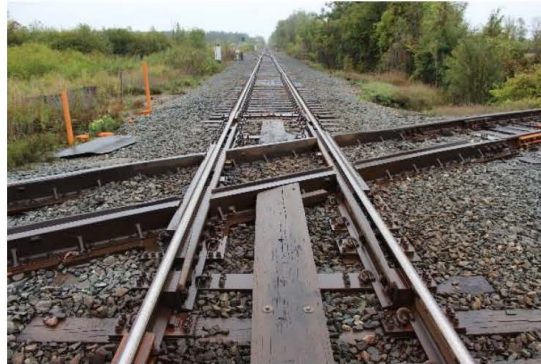
Figure 2-10: Diamond between BCRY and CP
