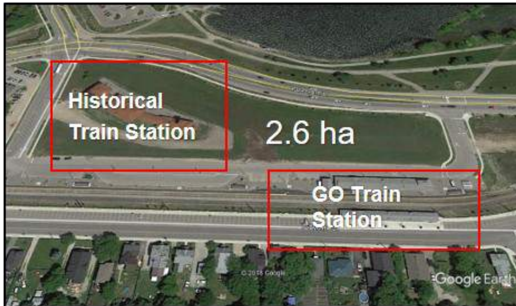
Figure 4-8 City of Barrie Allandale Waterfront GO Station Site
