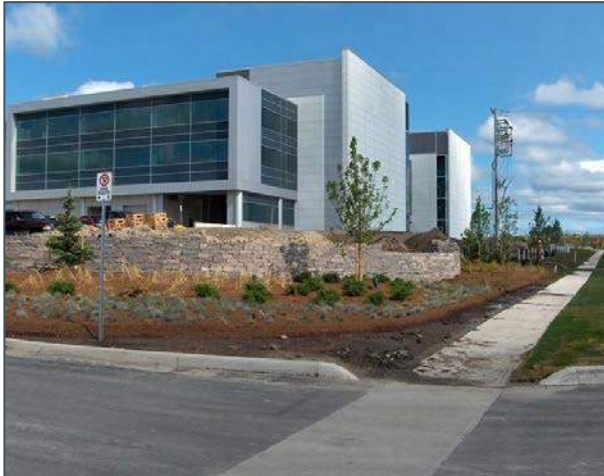
Bank of Montreal Barrie Computing Customer Data Disaster Recovery Centre Centre (Data Centre); 50 Reid Drive GFA: 30,660 sq.m (330,000 sq.ft.) Land Area: 10 ha (25 acres)
