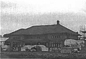
285 Bradford Street "Allandale Train Station" By-Law 2009-144 Aug10/09
