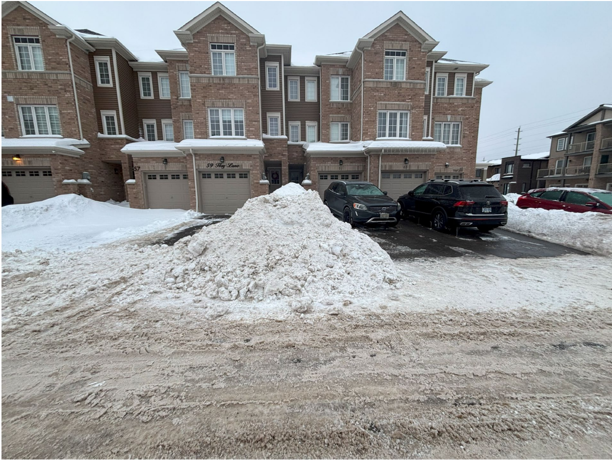
This photo is another example of a 4.5 metre lot frontage with insufficient snow storage. These units have slightly longer driveways as the sidewalk is not located on this side of the street.
