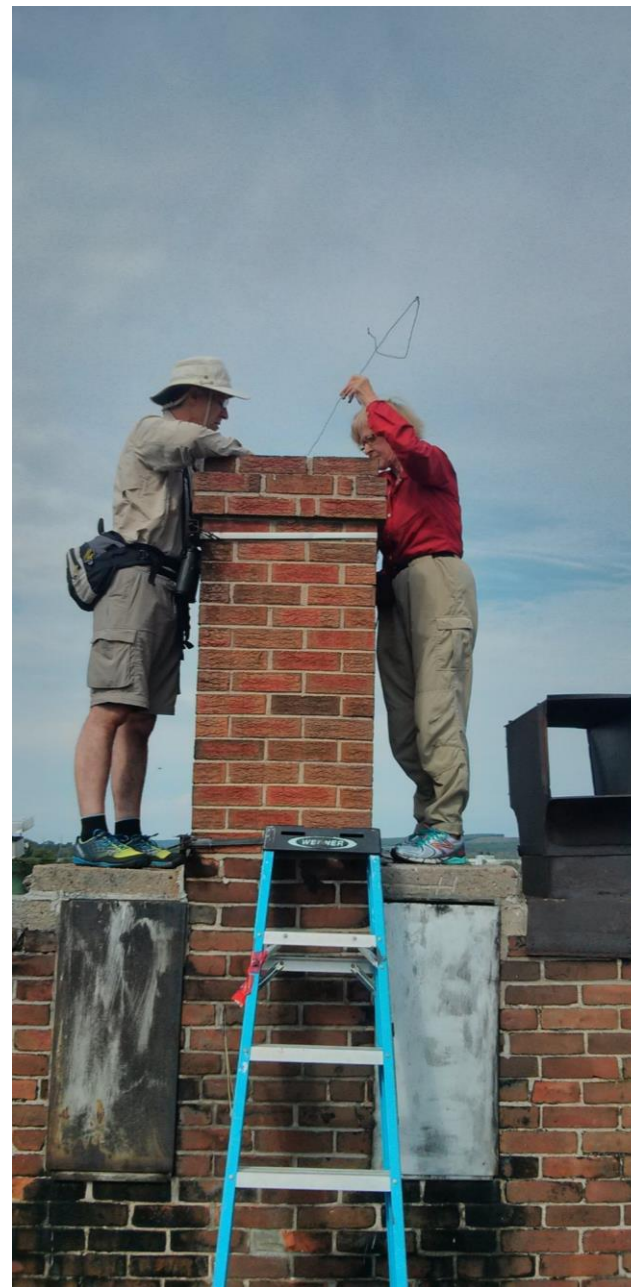
Unity Christian High School chimney and camera (putting temperature monitor in)
