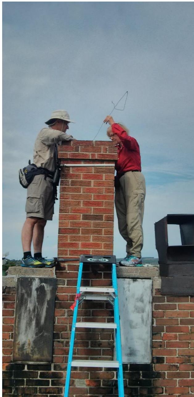
Unity Christian High School chimney – installing temperature data logger
