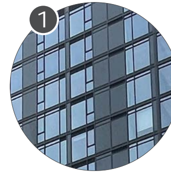
1 Window Wall System with Insulated Glazing
