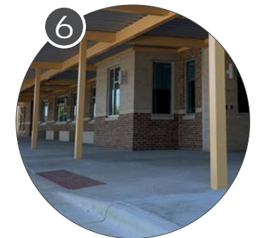
6 Accessible Semi-covered Walkways
