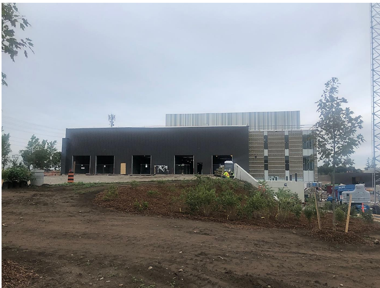
South Elevation of Building 'A' – September 16, 2019
