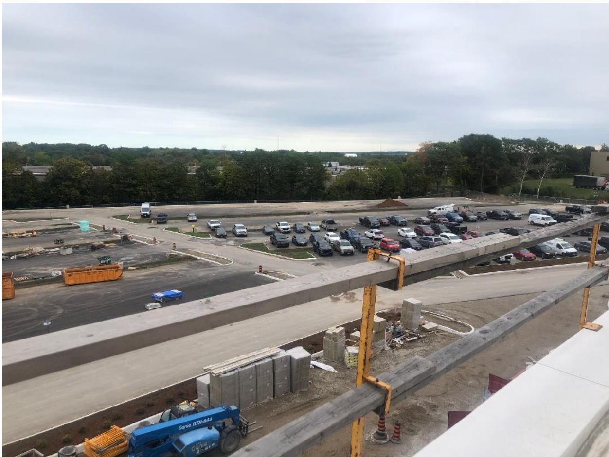
Parking Lot and Earthworks in Progress – September 16, 2019
