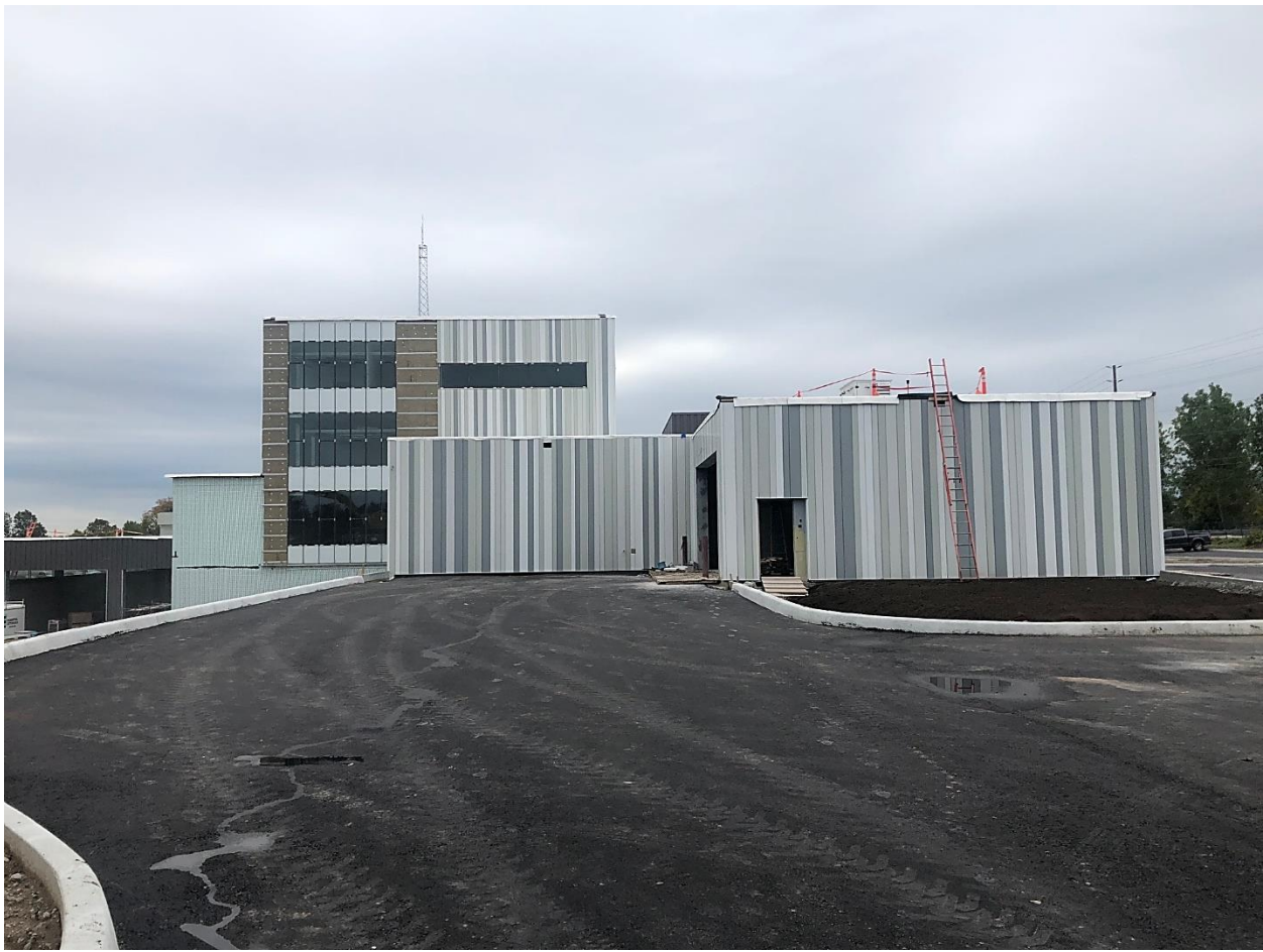
North Elevation of Building 'A' – September 16, 2019
