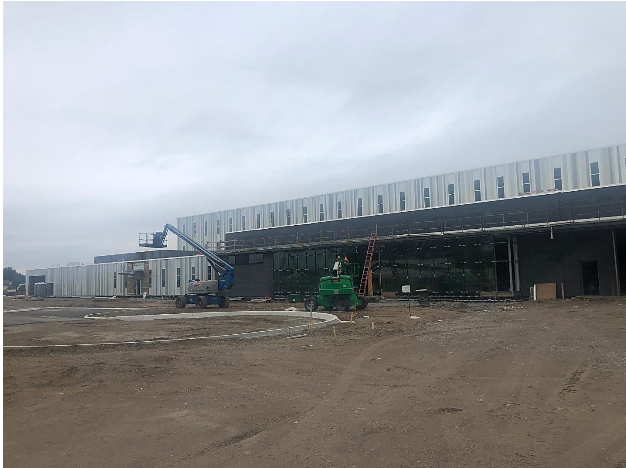
Partial West Elevation of Building 'A' (along Fairview Road) – September 16, 2019
