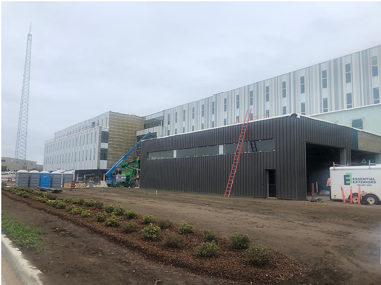
Partial West Elevation of Building 'A' Progress – September 16, 2019
