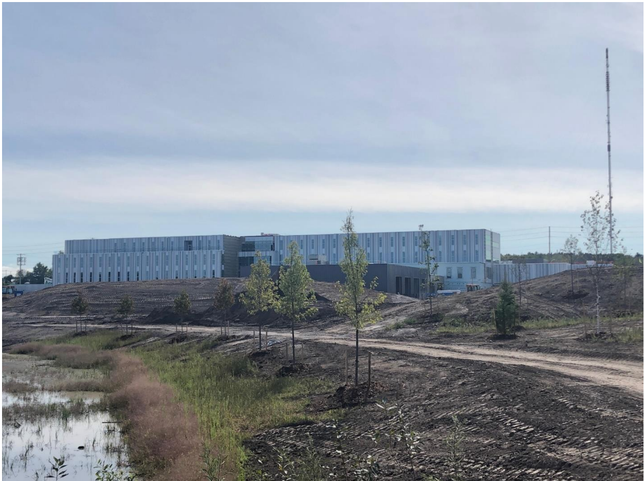
East Elevation of Building 'A' and Landscaping – September 16, 2019
