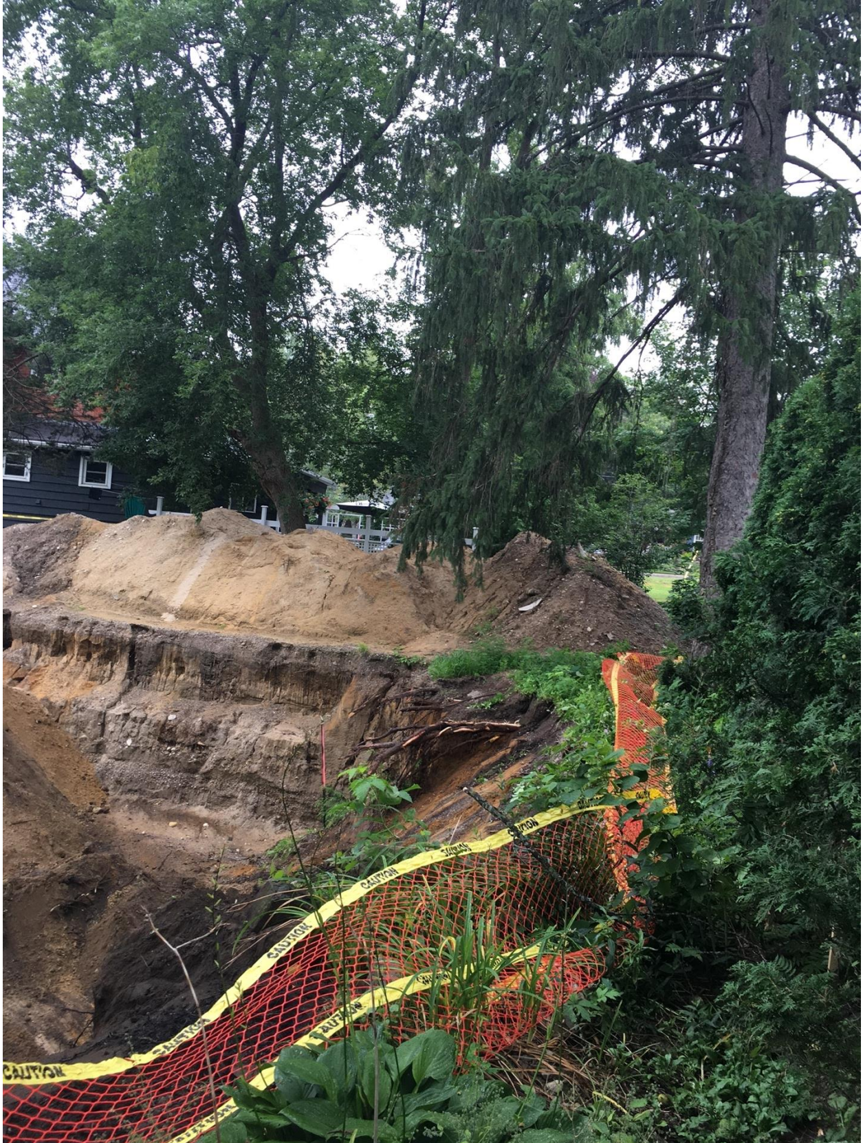
Aug 17 Severed roots of spruce, illegal vertical pit walls, fencing flattened
