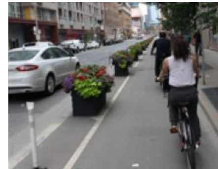
Bicycle Lane Physically Separated by Bollards, Markham
