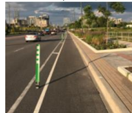
Bicycle Lane Physically Separated by Bollards, Markham
