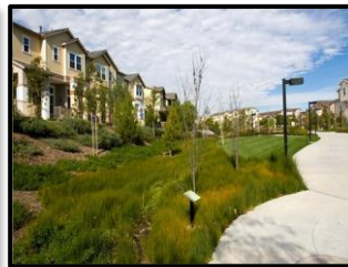
Bioretention Cell
