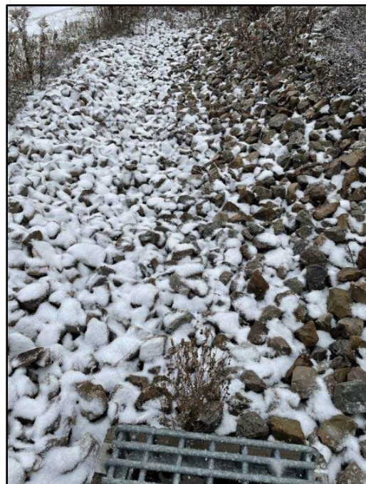
Image 12: Pond 2 West Conveyance Channel, view south
