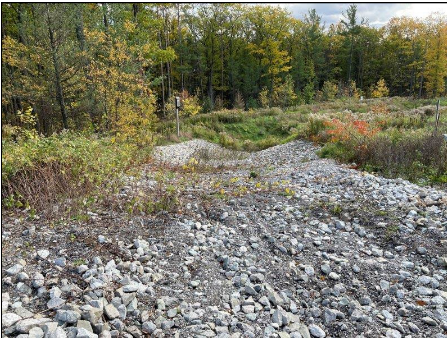
Image 27: Pond 5 Conveyance Channel
