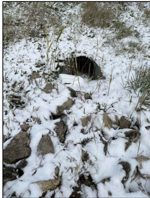
Image 63: Compost Pond Southwest Culvert Inlet
