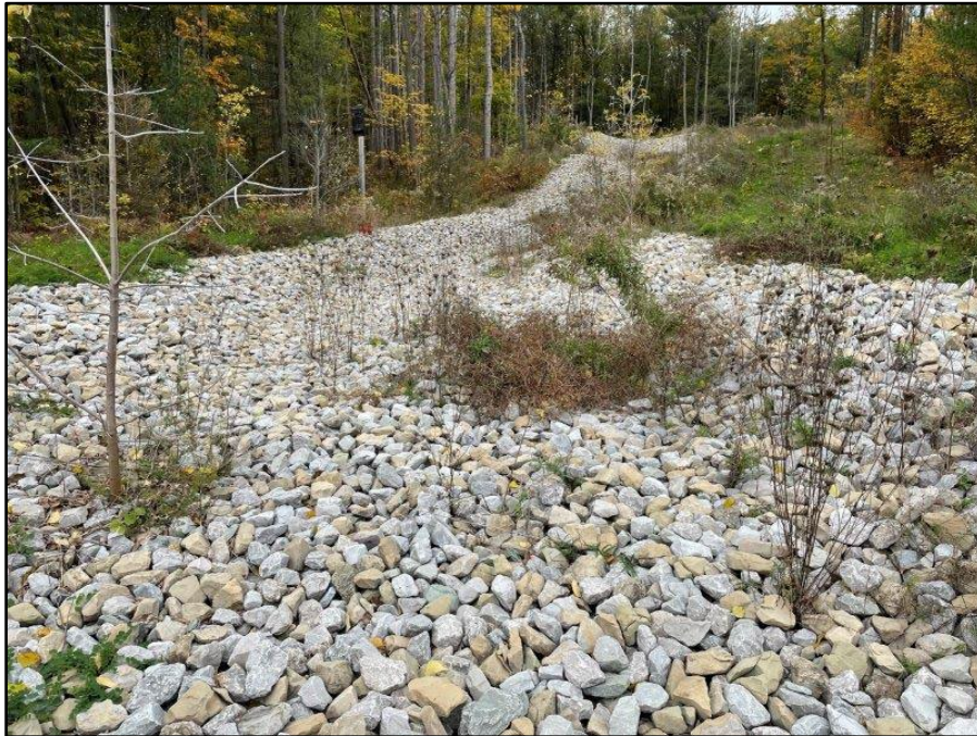
Image 43: Pond 8 West Conveyance Swale, view northwest
