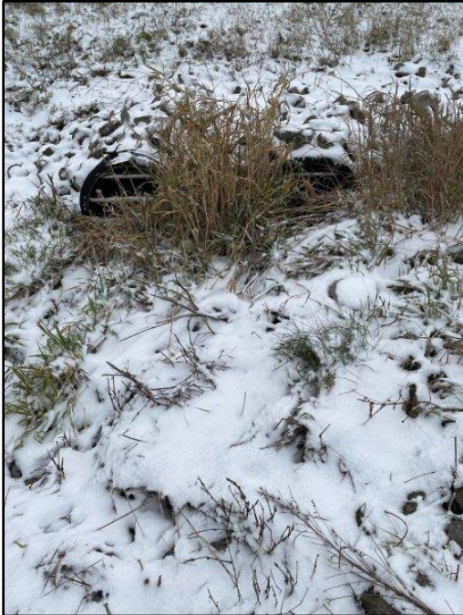
Image 64: Compost Pond Northwest Culvert Inlets
