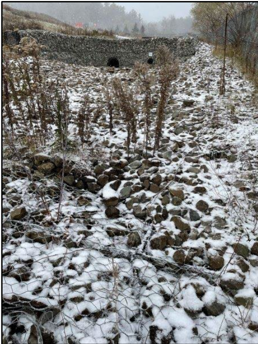
Image 17: Pond 2 Plunge Pool Discharge Channel to Dyments Creek
