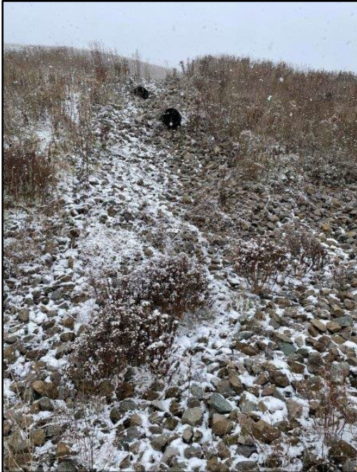
Image 9: Pond 1 Discharge and Overflow Channel
