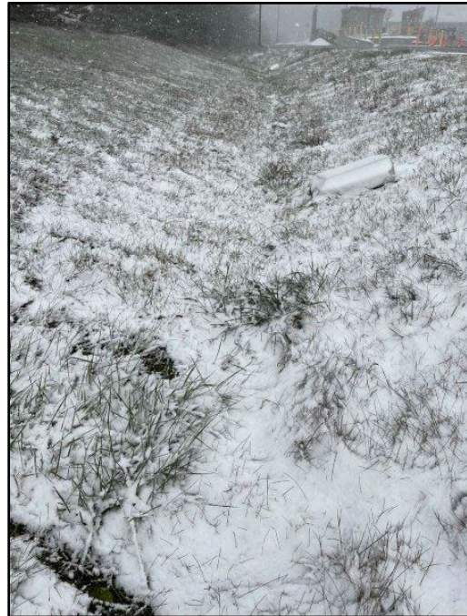
Image 111: North Ditch, view northeast
