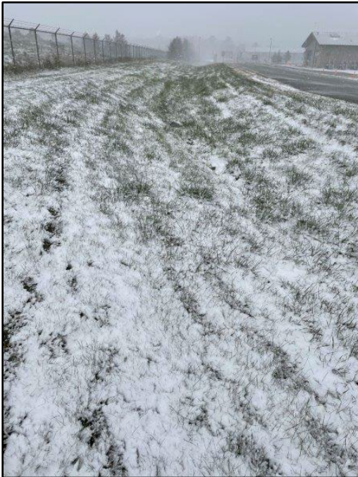
Image 109: North Ditch, view northeast
