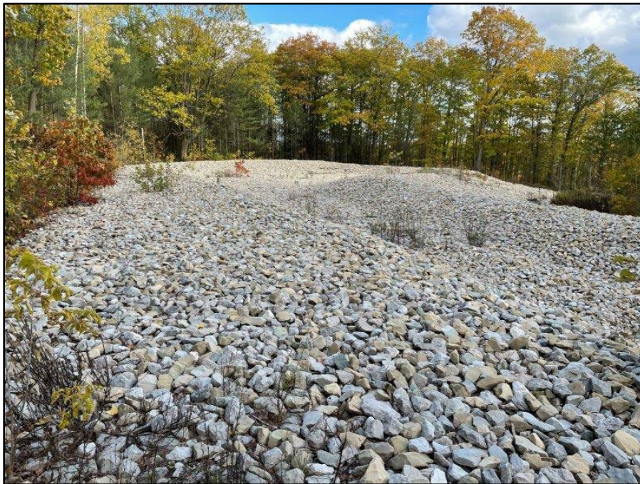
Image 57: Final Outfall Channel Flow Spreader to Edgehill Drive, view east
