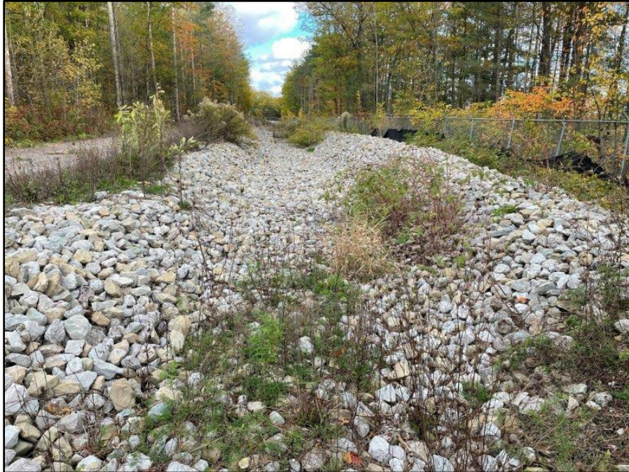
Image 52: Final Outfall Channel to Edgehill Drive, view east
