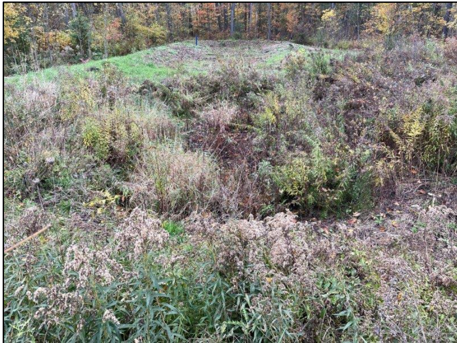
Image 19: Pond 3 Forebay, view southwest
