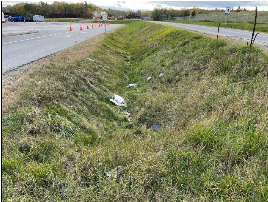
Image 106: Ditch North of Household Hazardous Waste and Commodities, view southwest
