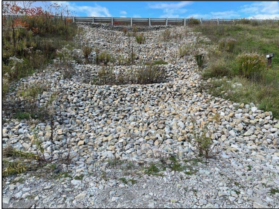
Image 36: Pond 7 Conveyance Channel
