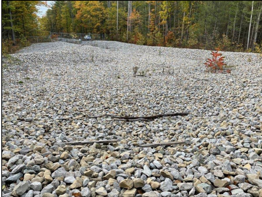
Image 56: Final Outfall Channel Flow Spreader to Edgehill Drive, view west
