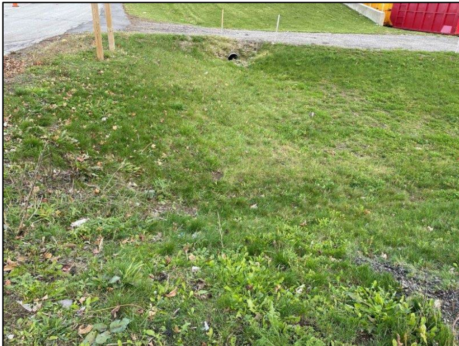
Image 99: Culvert Outlet Southeast of Waste & Recycling Depot
