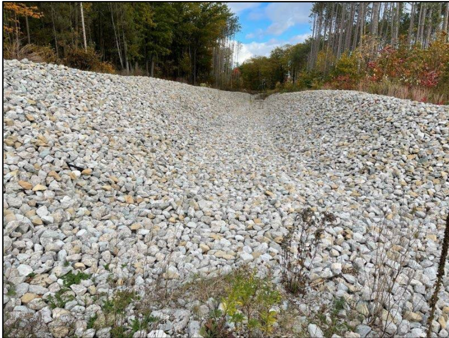
Image 50: Final Outfall Channel to Edgehill Drive, view east
