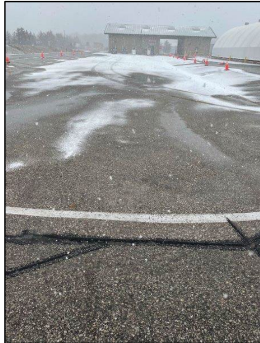
Image 86: Finished Compost Storage
