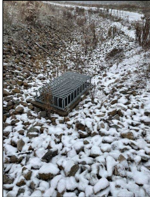
Image 11: Pond 2 West Conveyance Channel and Ditch Inlet Structure, view north
