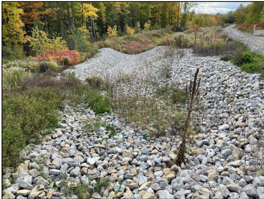
Image 31: Pond 6 Conveyance Channel
