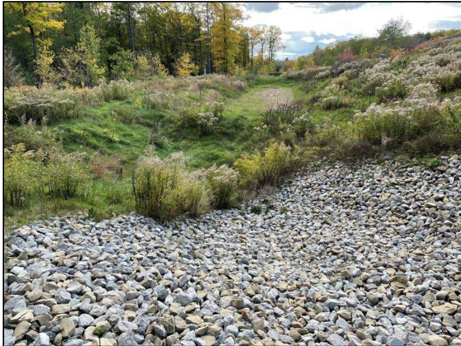
Image 28: Pond 5 Forebay, view southwest
