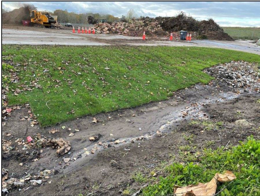
Image 96: New Sod Installed in West Ditch, view west
