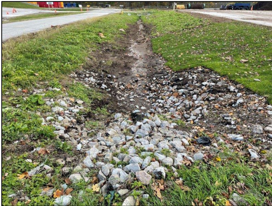
Image 97: West Ditch, view southeast
