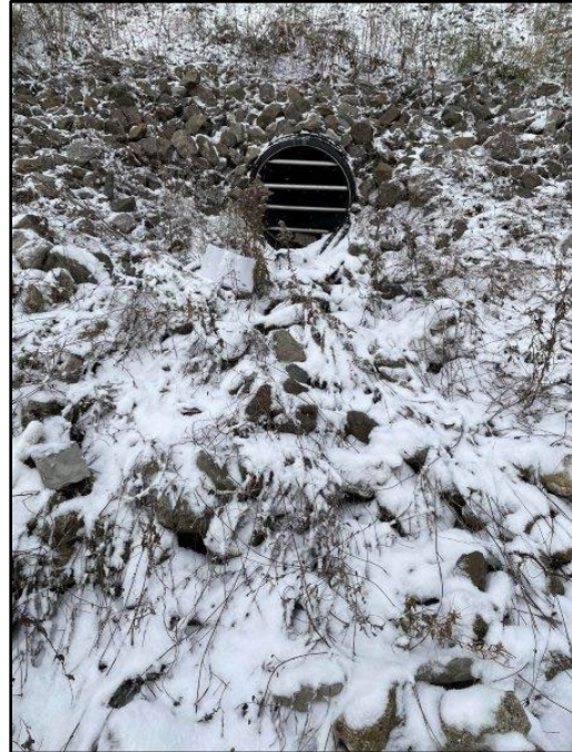
Image 65: Compost Pond Northeast Culvert Inlet
