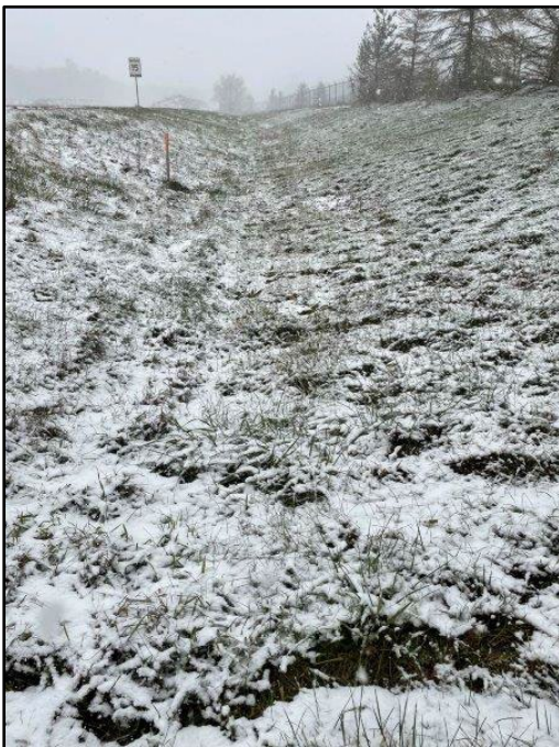
Image 110: North Ditch, view west
