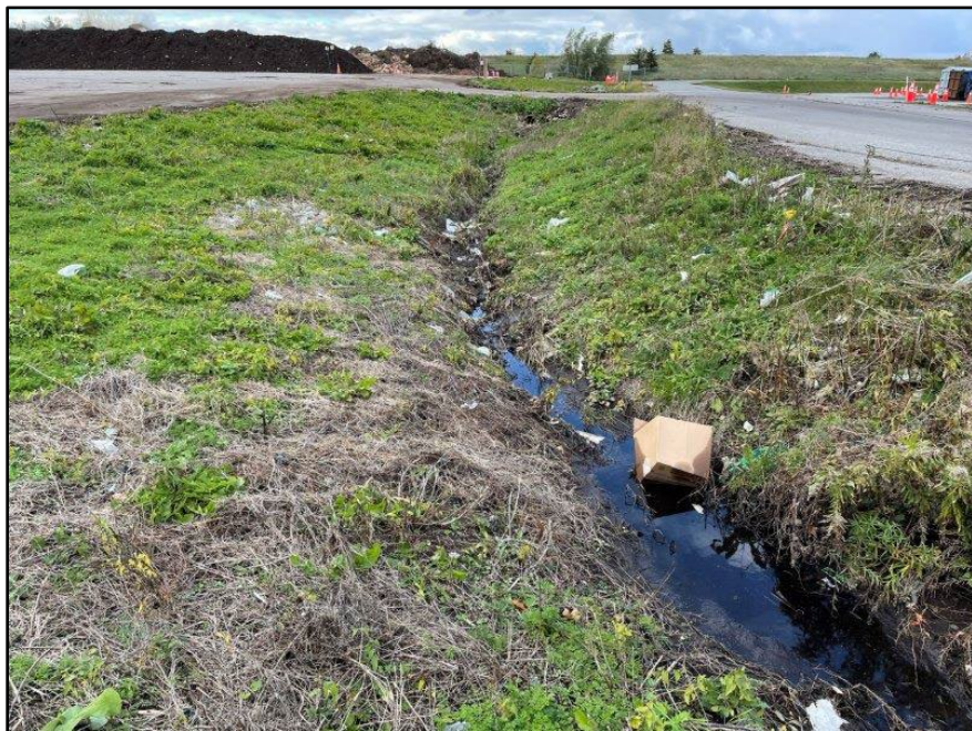
Image 67: Compost Pond Conveyance Ditch, view northwest
