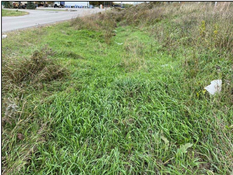
Image 73: North Access Road Ditch, view northeast
