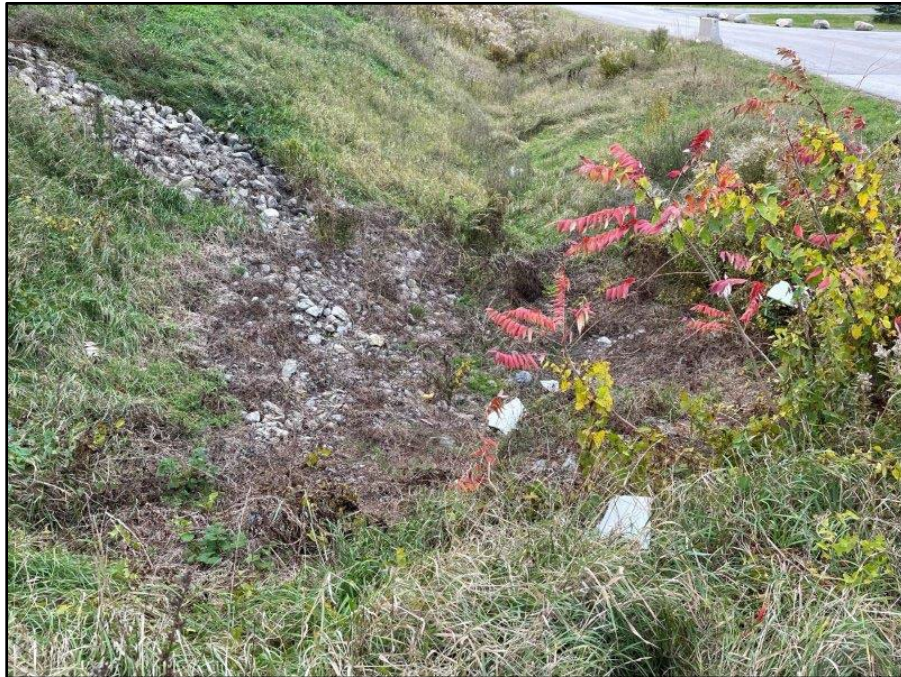
Image 74: North Access Road Ditch, view southwest
