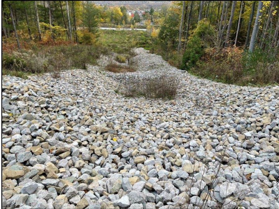
Image 42: Pond 8 West Conveyance Swale
