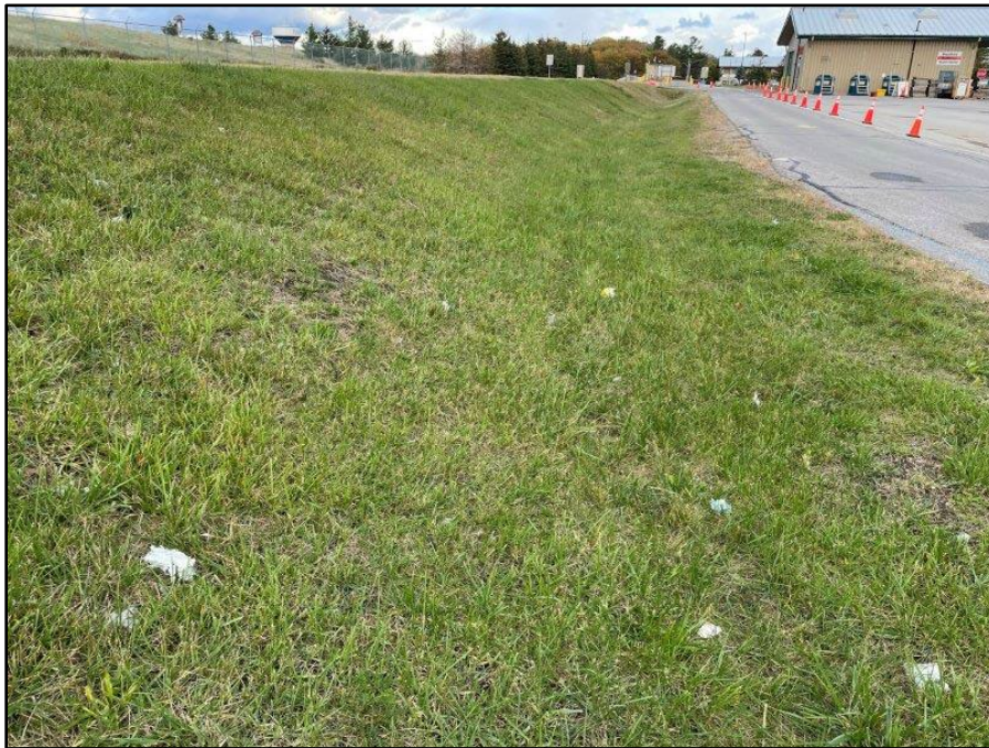
Image 105: Ditch West of Household Hazardous Waste and Commodities, view northeast
