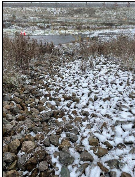
Image 8: Pond 1 Discharge and Overflow Channel
