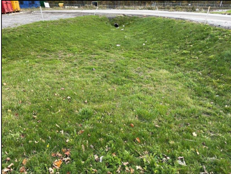
Image 100: Culvert Inlet Southeast of Waste and Recycling Depot
