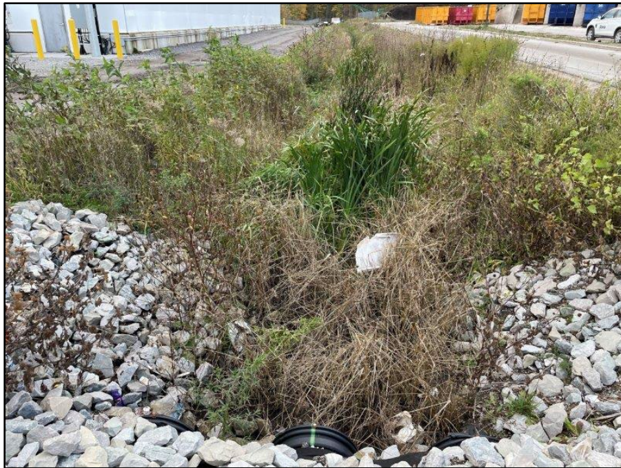
Image 69: Compost Pond Conveyance Ditch at West Access Road, view southwest
