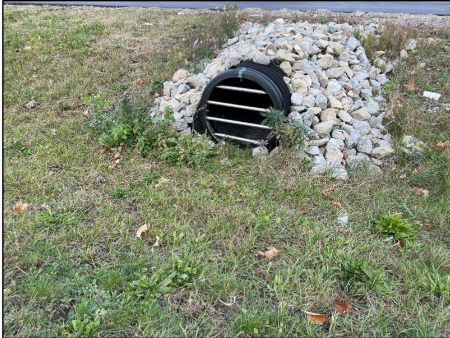
Image 102: Culvert Outlet in Ditch West of Waste and Recycling Depot
