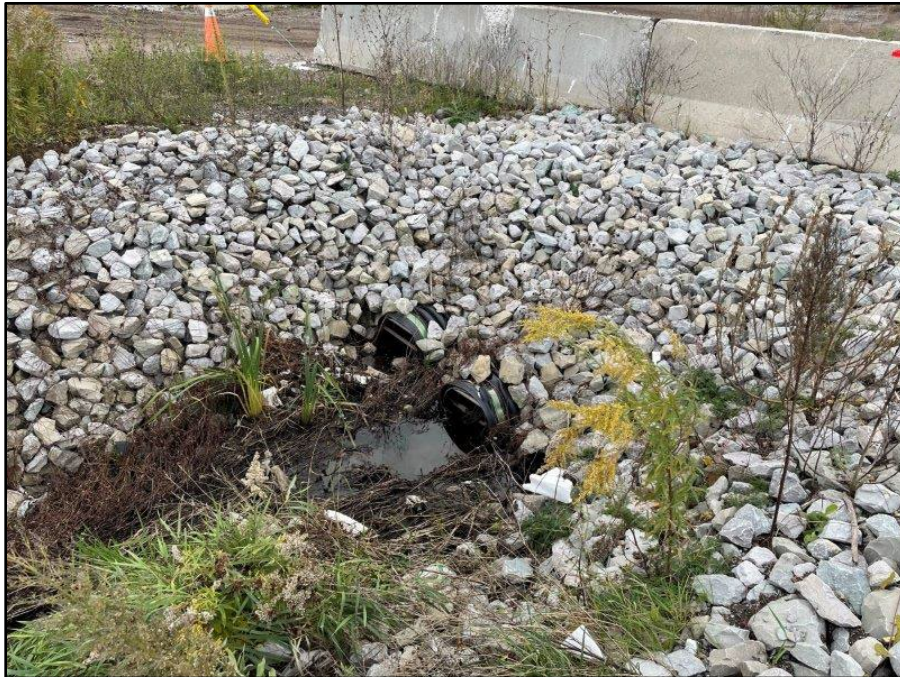
Image 70: West Access Road Culvert Outlets
