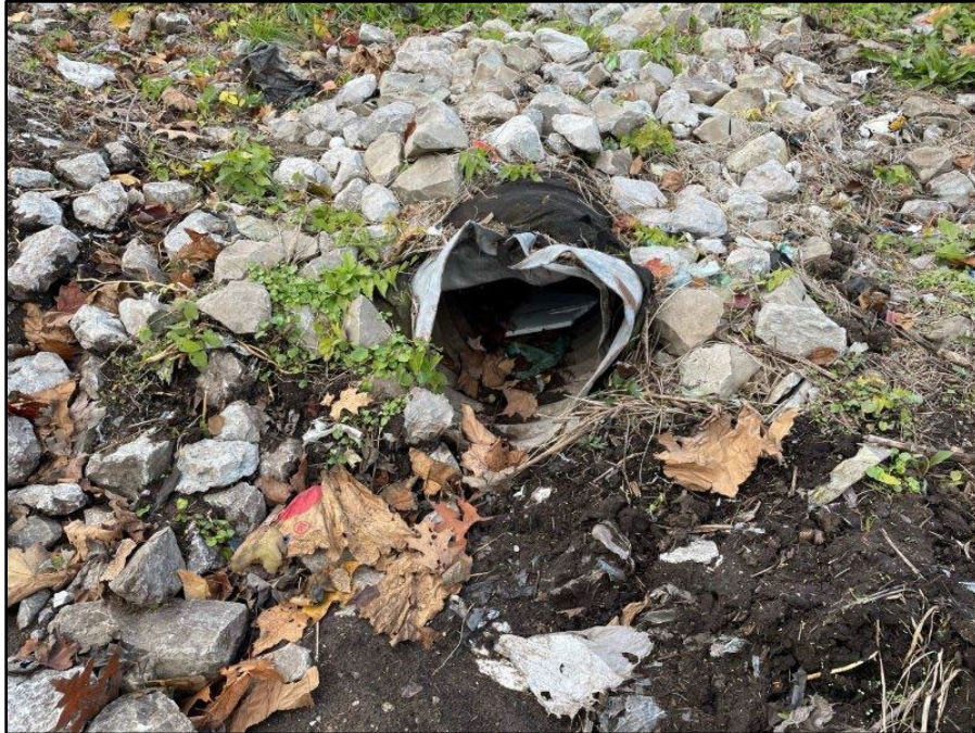
Image 98: West Ditch Culvert Inlet at North Entrance to Compost Pad
