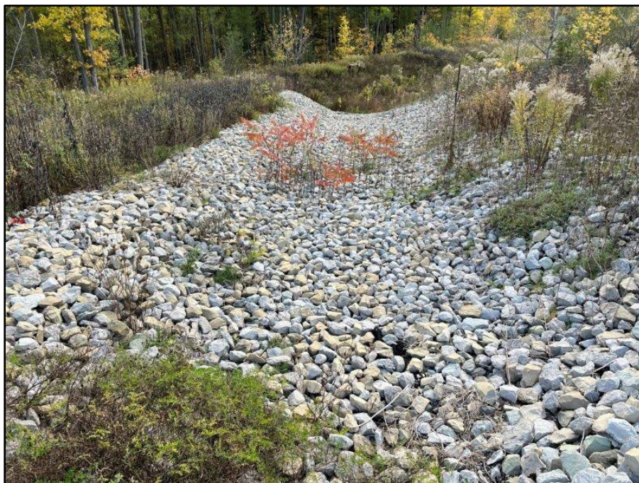
Image 37: Pond 7 Conveyance Channel
