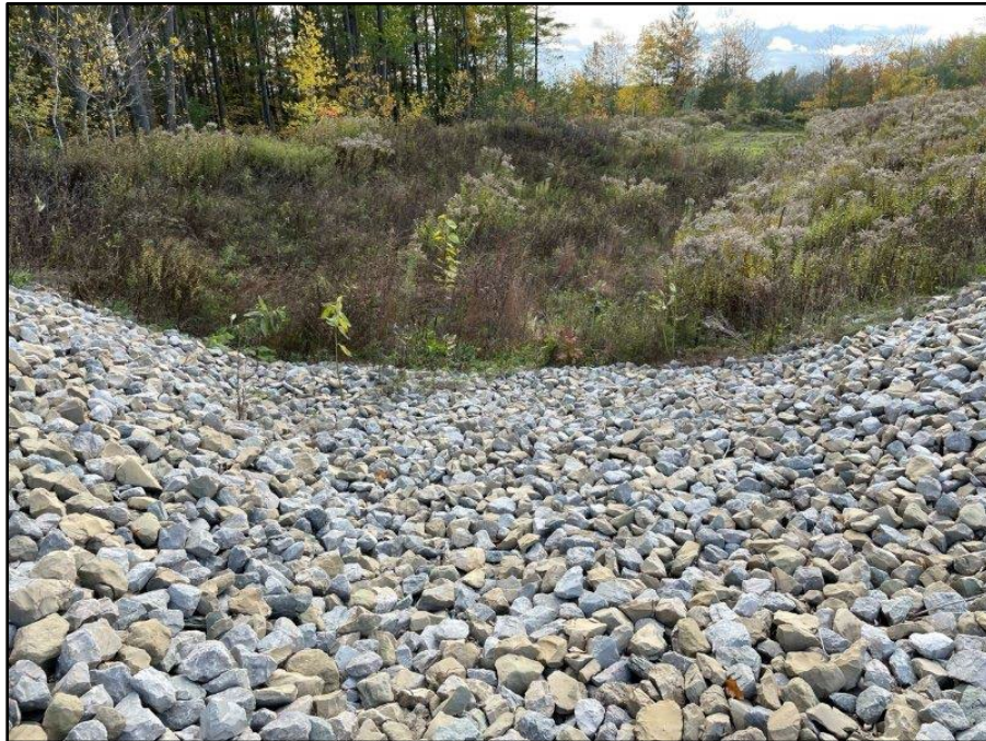
Image 38: Pond 7 Forebay, view southwest
