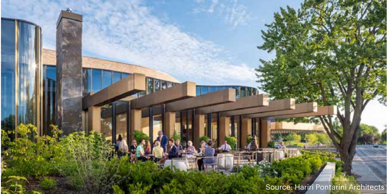
Source: Hariri Pontarini Architects The newly opened 600-seat Tom Patterson Theatre in Stratford, ON, focuses on expanded patron experience, including publicly accessible gardens and a terrace with seating.
