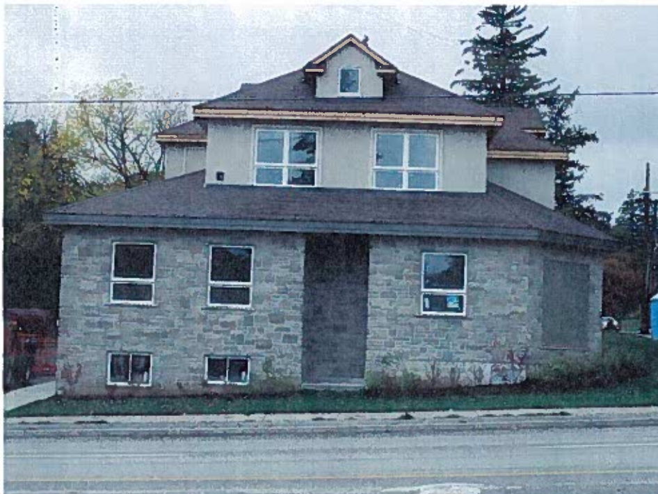
Under construction: - Looking west from Bayfield Street (source applicant)
