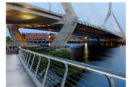
North Bank Bridge Park Boston, MA
