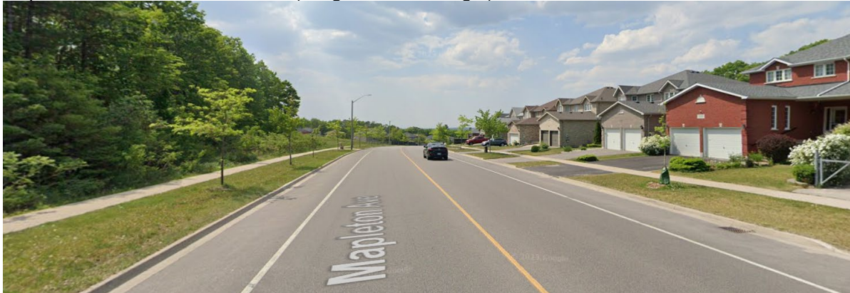
Mapleton Avenue Urban Shoulder (image source: Google)
