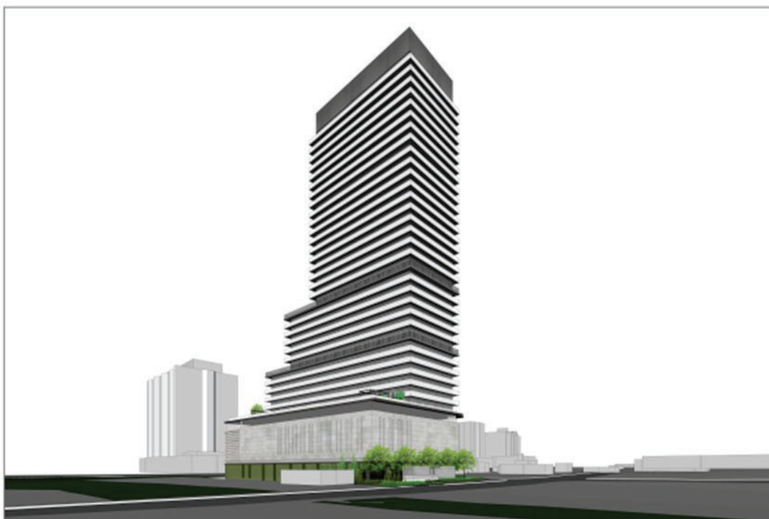
2 NORTH WEST CORNER
