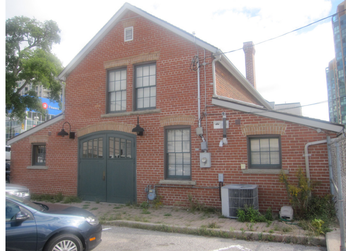
◀ Figure 4.3 Back, west elevation
