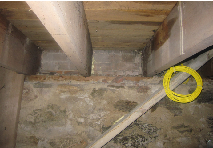
◀ Figure 4.10 Crawlspace joists and wall at north wall
