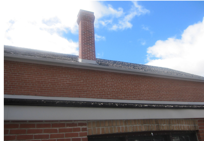
◀ Figure 4.15 North Chimney
