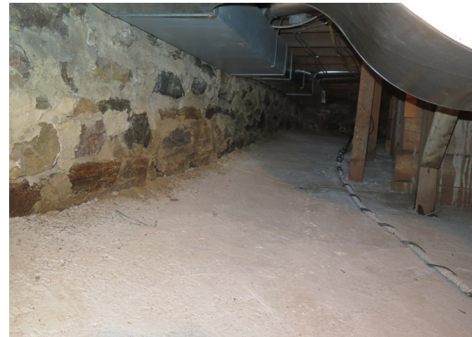
◀ Figure 4.8 Crawlspace looking east
