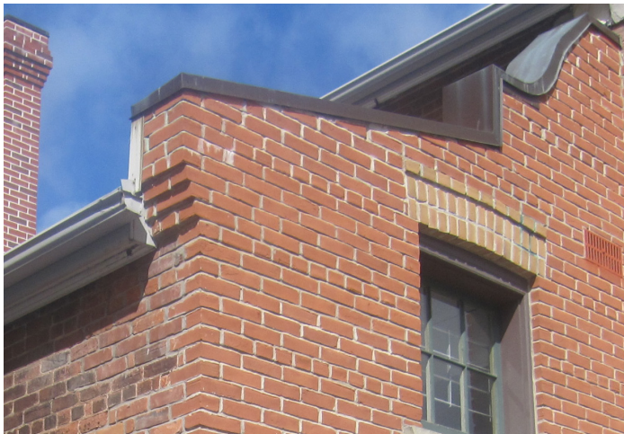
◀ Figure 4.14 Flashing at parapet and fascia
