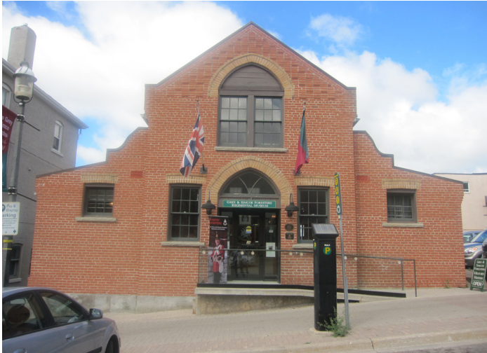
◀ Figure 4.1 Front, east elevation
