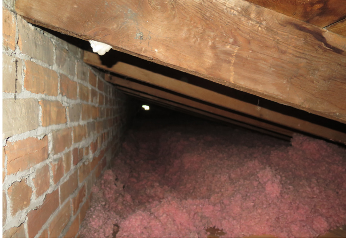
◀ Figure 4.17 South Attic
