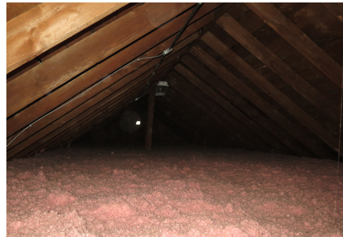
◀ Figure 4.16 Main Attic
