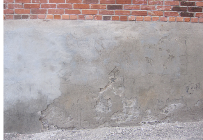
◀ Figure 4.11 South side parging
