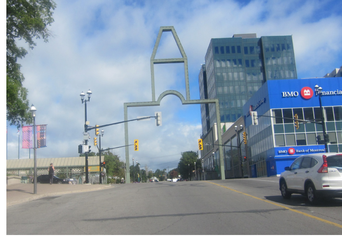
◀ Figure 5.7 Historic City Hall Arch (north west view)
