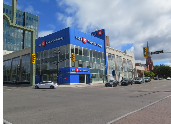
◀ Figure 5.3 North East Corner
