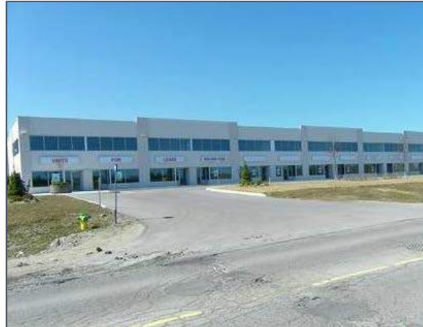
Multi-Tenant Industrial Building (2-storey) 353 Saunders Road GFA: 4,650 sq.m (50,000 sq.ft.) Land Area: 1 ha (2.5 acres)
