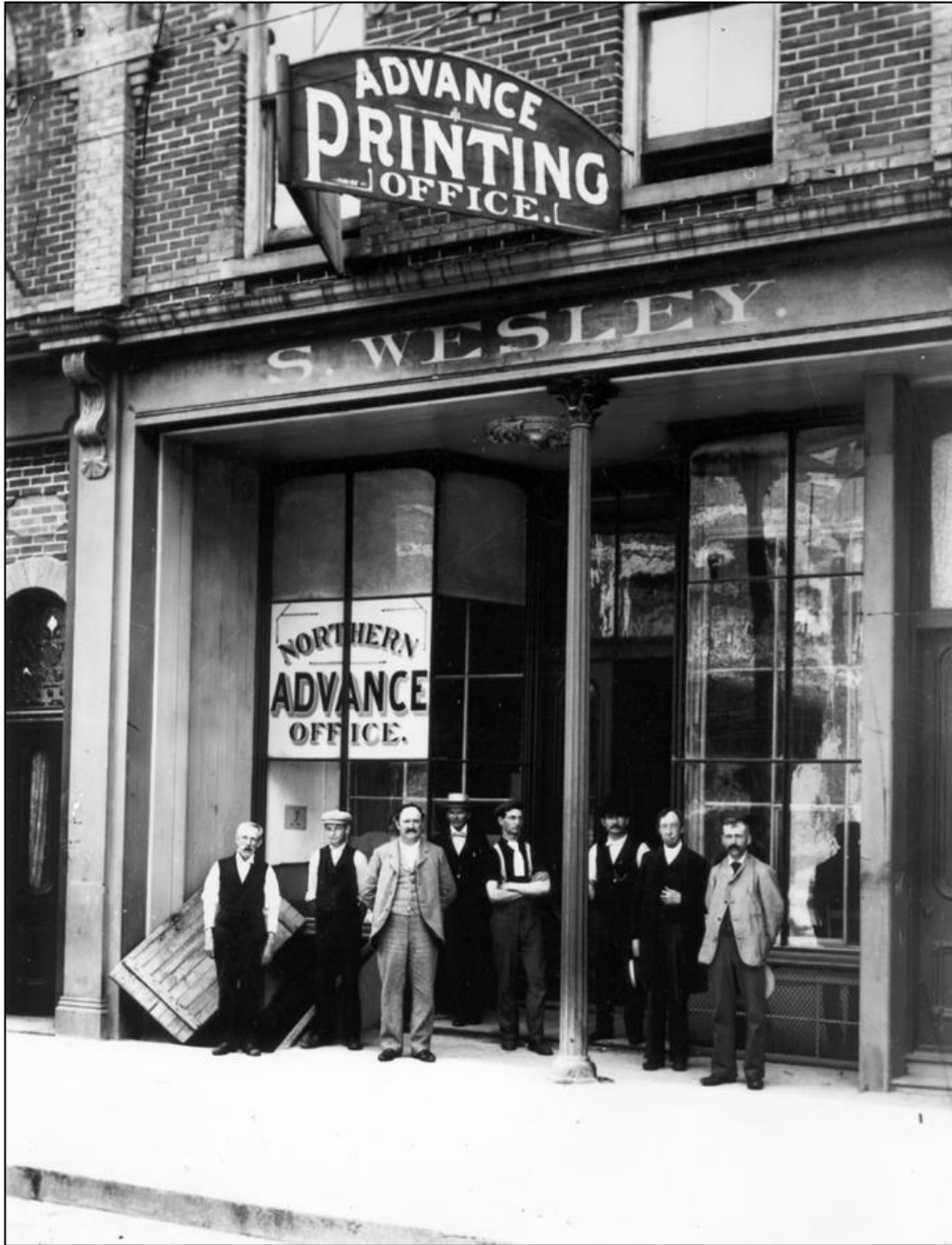
Figure 13: This photograph is undated but The “Cheap Boot and Shoe Store” building at 121-123 Dunlop owned by John Culverwell (shown) became the Northern Advance newspaper office in 1883. The upper level façade of this storefront matches No. 125-127 abutting on the left (east). Only the west (right) edge of No. 125-127 is in view and reveals art glass in the transom over an entranceway. (Photo: Simcoe County Archives)
