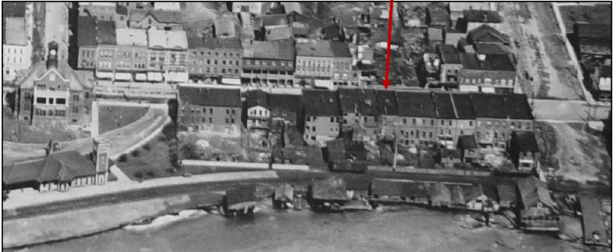
Figure 21: Aerial view, c.1927. Arrow indicates the location of 125-127 Dunlop Street East. Note the firewalls rising above the roof creating parapets between each subgrouping of stores. (Photo: Simcoe County Archives)
