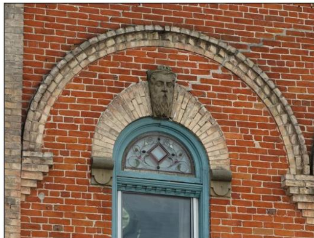
Figure 29: Window treatment showing the semicircular shaped opening, radiating brick voussoir (surround) with the portrait head keystone, terminating in terracotta stone (or stone) ends; with a tri-layer arch with corbelled plinth ends above, November 2021. The original window sashes have been replaced with a transom with art glass and a moulded frame. The lower sashes are modern.
