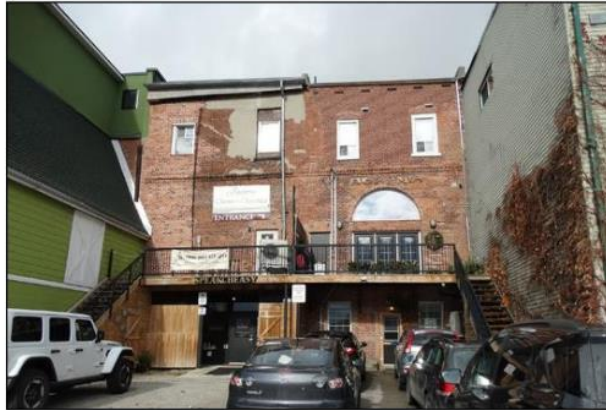
Figure 32: Above and Below: The rear of 125-127 Dunlop Street East is the red brick, three storey structure to the right, November 2021. The large, semicircular window opening was added by the current owner. The stair access, decking, and entrance on the left to the upper level are recent.
