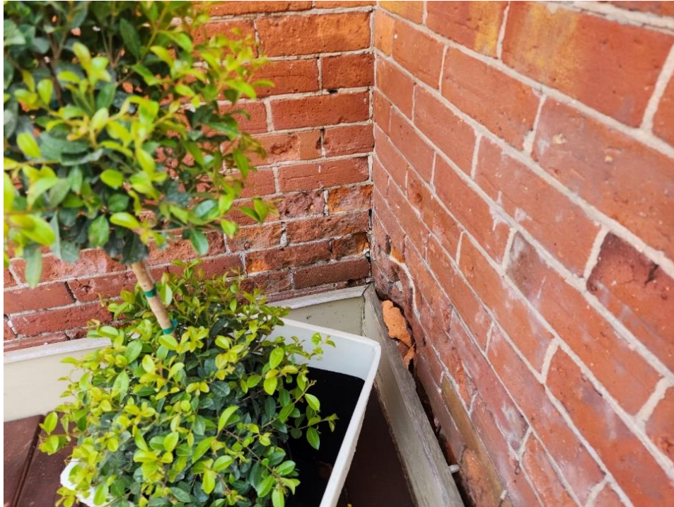
Image 2 – Photograph of one area where brick is to be repointed.
