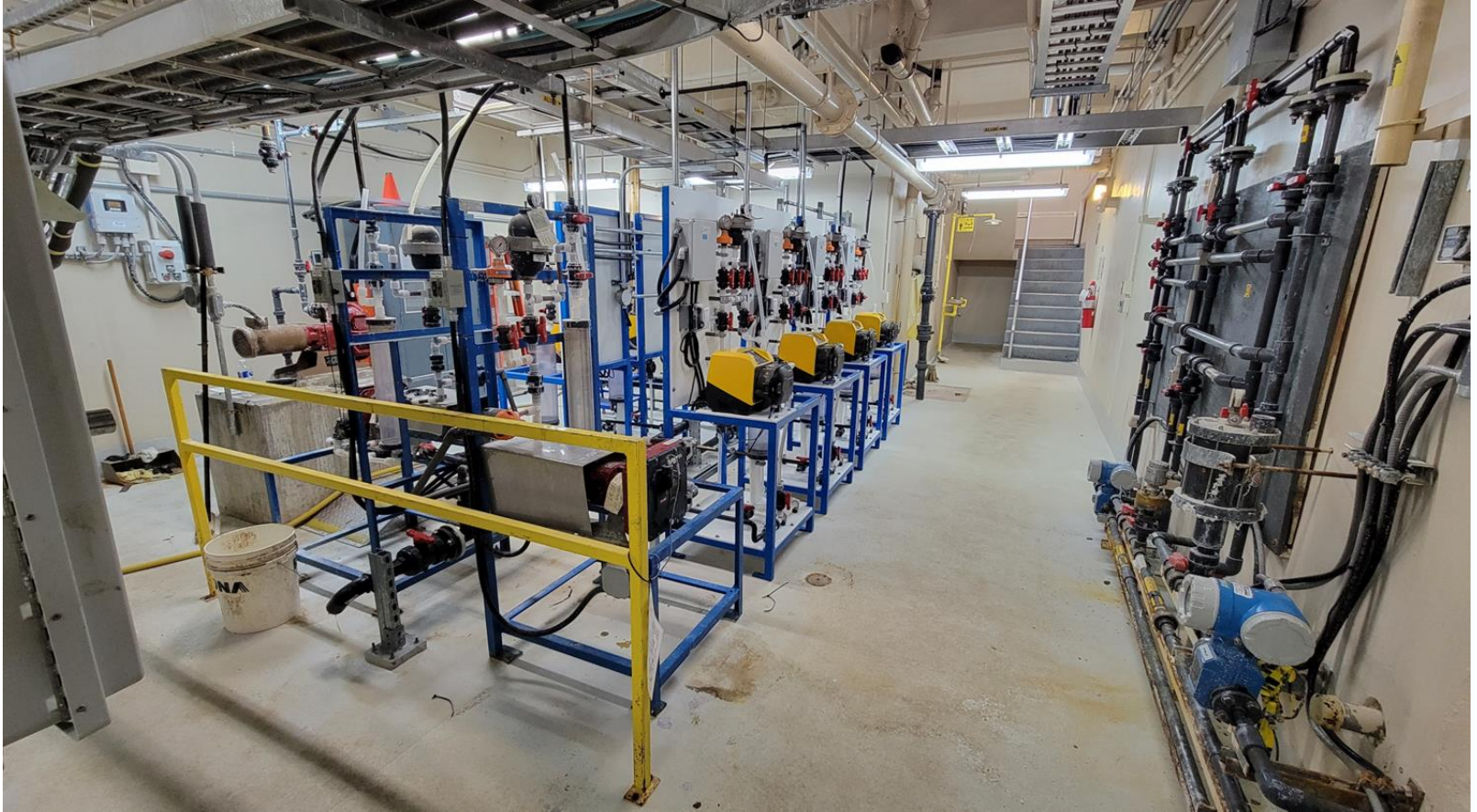
Alum Dosing at Wastewater Treatment Facility
