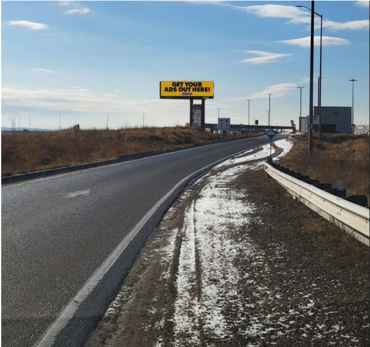
VIEW SOUTHBOUND RAMP TO ONroute, APPROXIMATELY 150 METRES FROM SIGN
