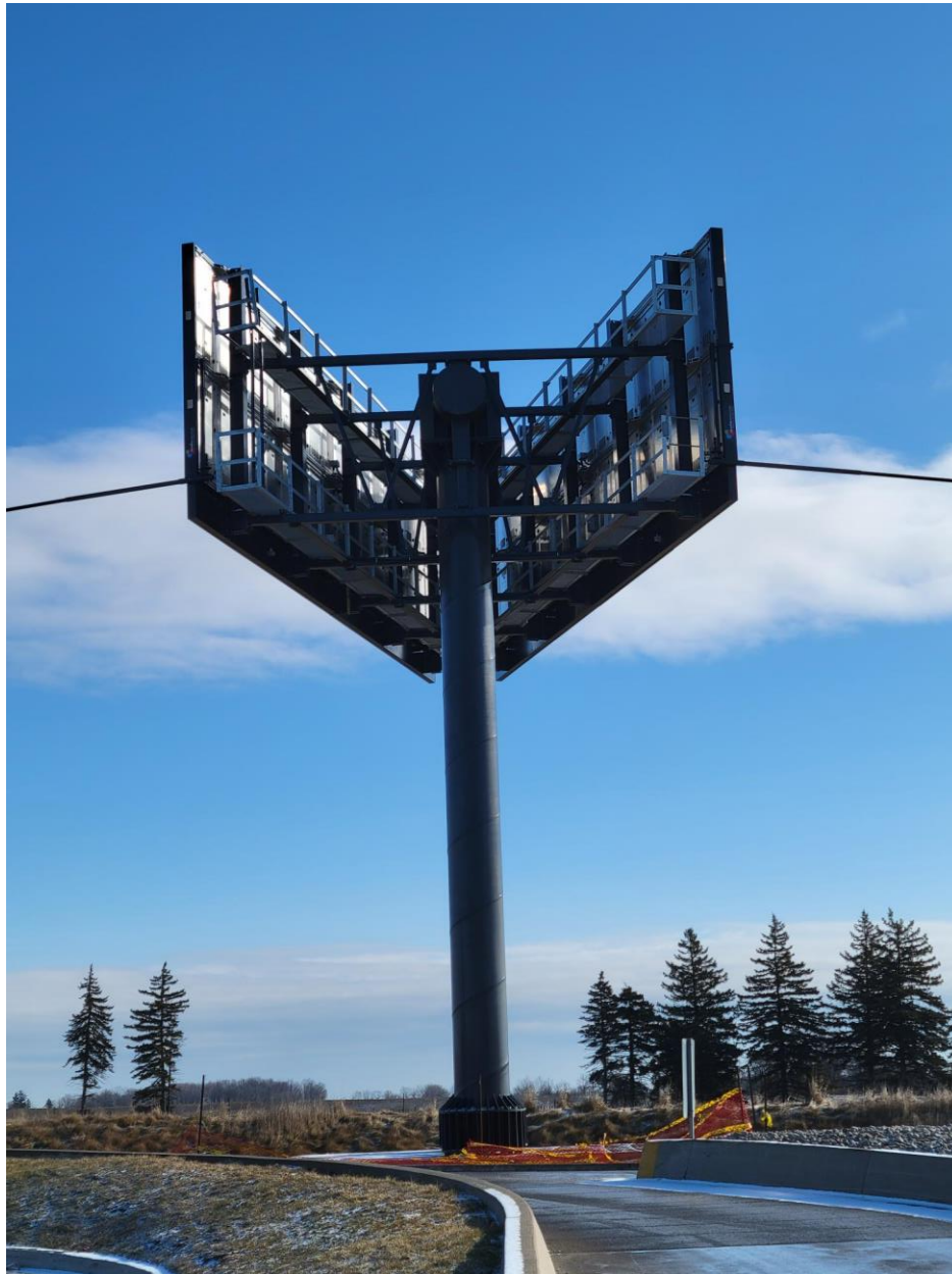
VIEW FROM REAR OF THE SIGN, APPROXIMATELY 35 METRES FROM SIGN
