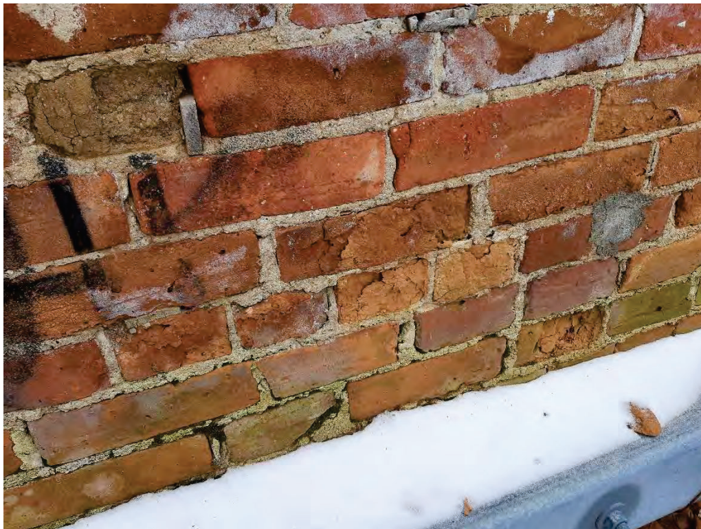
Photograph No. 11 – Isolated spalling observed on the brick surface in the interior wythe of brick.
