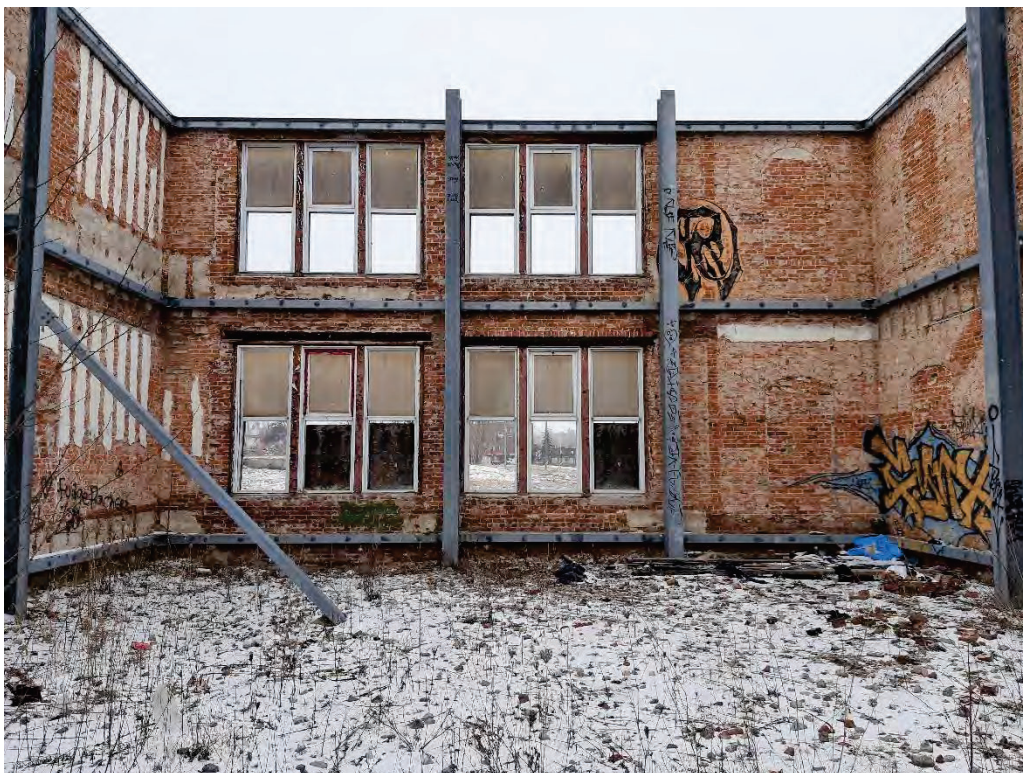
Photograph No. 2 – Temporary structural steel shoring facing the North Elevation in the Interior.
