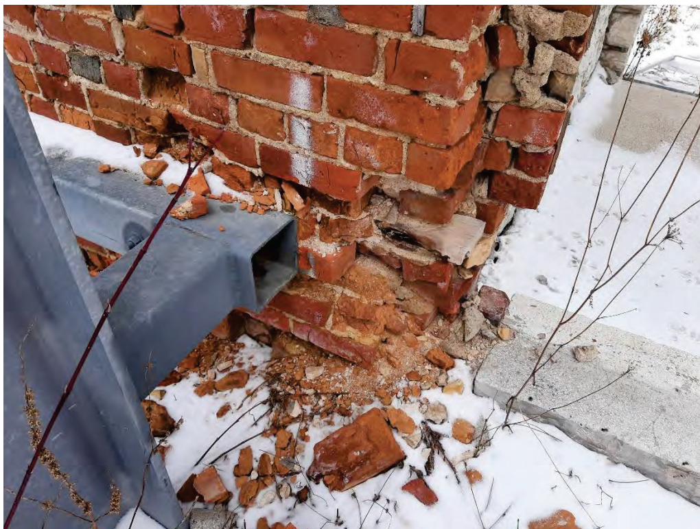
Photograph No. 10 – Deteriorated bricks at the bottom four courses at the former front opening.
