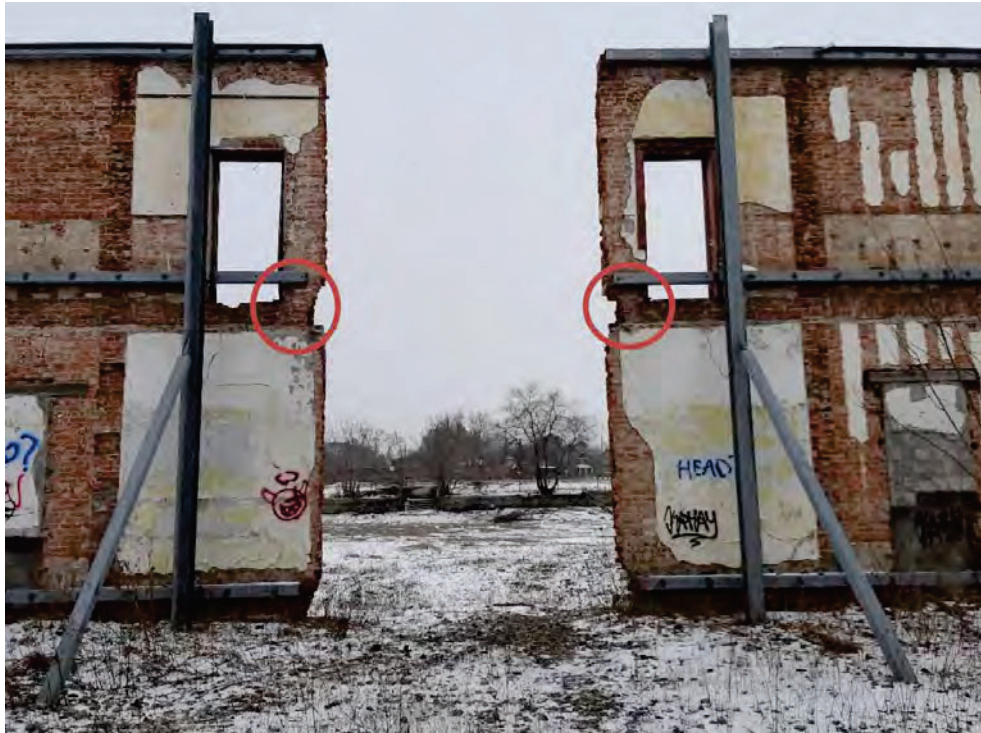
Figure 1: View of west wall opening with cracks showing under sills (source: MTE Consultants, 2024)
