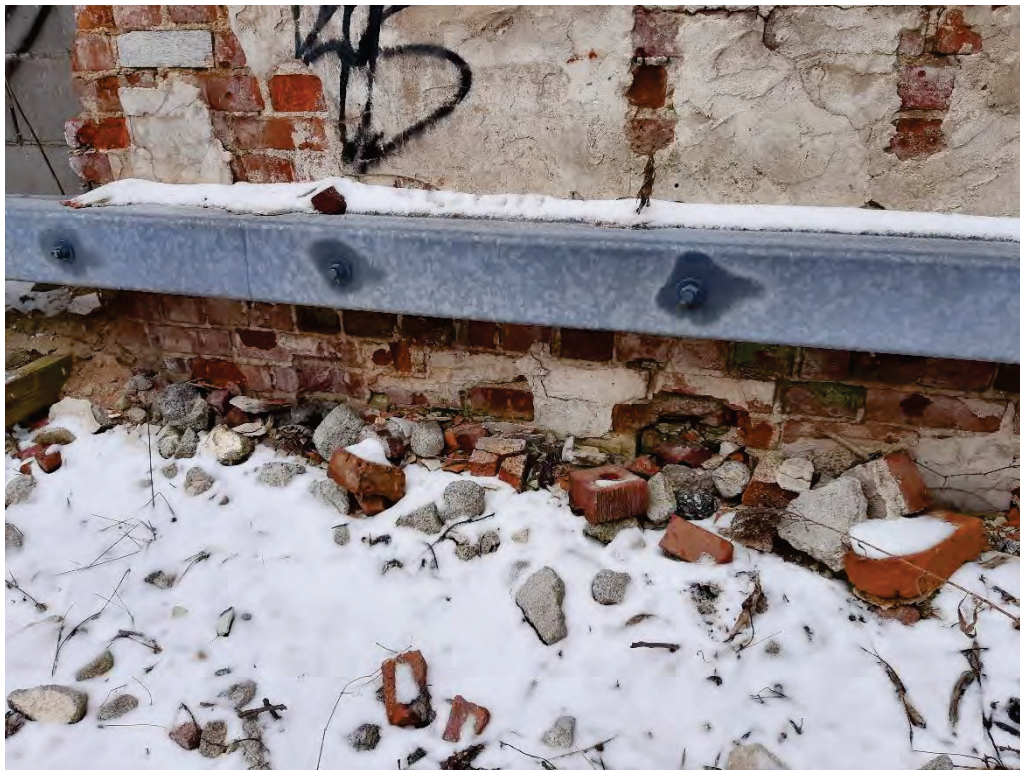
Photograph No. 9 – Deterioration of bottom four courses of bricks in the interior wythe.
