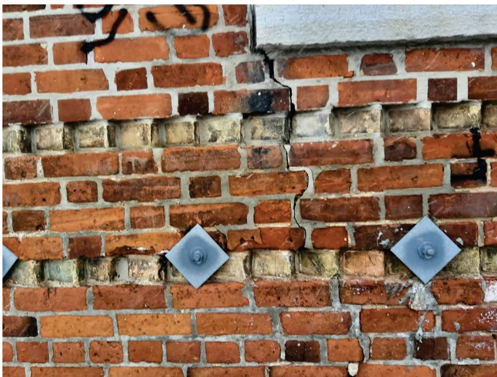
Photograph No. 12 – Some isolated step cracking noted in the brick on the exterior wythe.
