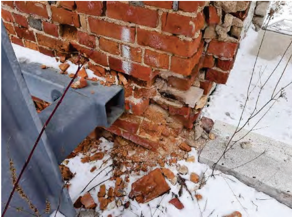
Figure 2: View of deteriorated bricks at bottom four courses of former front opening (source: MTE Consultants, 2024)
