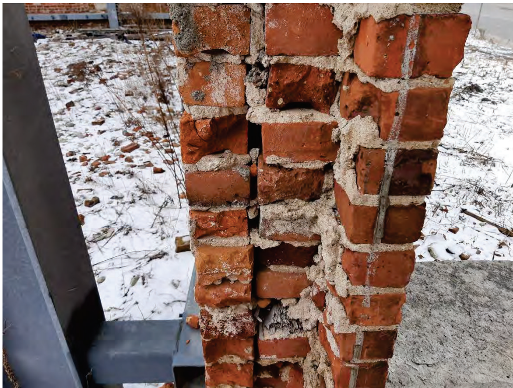
Photograph No. 8 – Cross section of the triple wythe wall.
