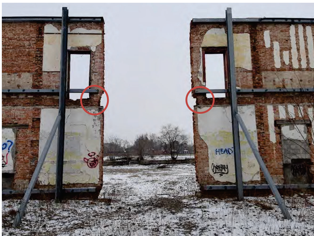
Photograph No. 6 – West wall opening with cracking showing under windows at small remaining cross-section.
