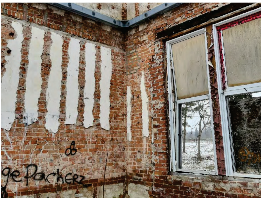
Photograph No. 14 – Some plaster on brick in the interior elevation remains. It appears that the removal process did not impact the face of the brick.
