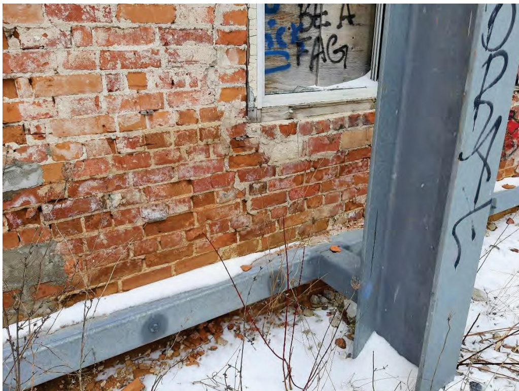
Photograph No. 3 – Interior view of the temporary shoring connection to the bottom of the wall at the interior.
