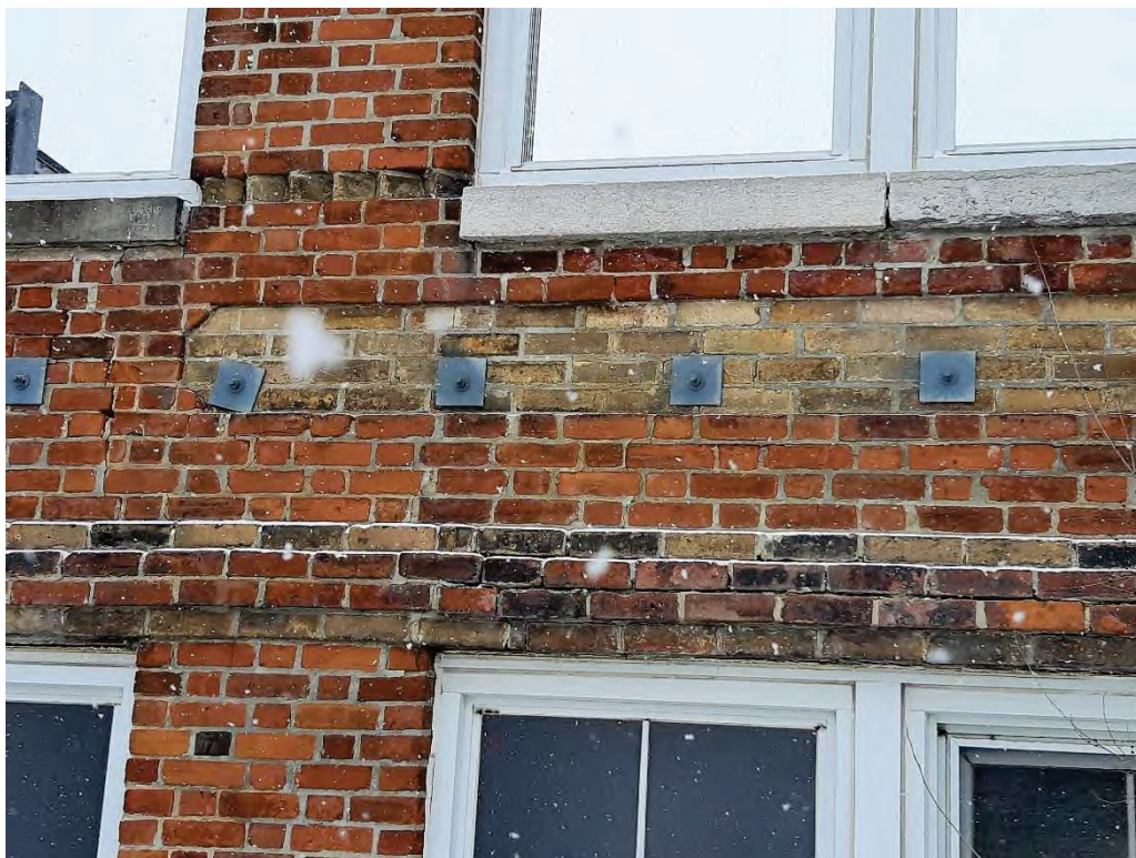
Photograph No. 4 – Through bolts at the mid height of the wall on the exterior south elevation.
