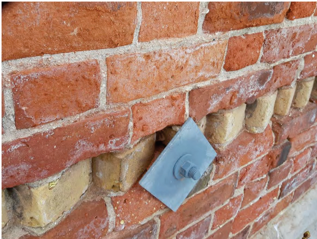
Photograph No. 5 – Close up of a through bolts.
