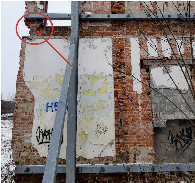
Photograph No. 7 – Cracking at the west wall below the windows.
