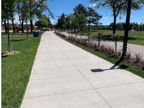
Concrete Walkway in Centennial Park
